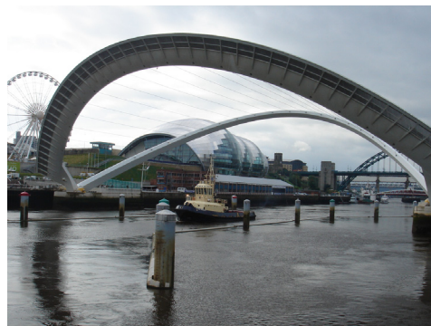
The Gateshead Millennium Bridge opening for a tug with the Ferris Wheel and Sage Music Centre in the background
