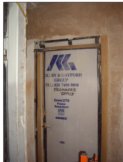
Past Master Willmot's door to the Engineers Office duly protected
