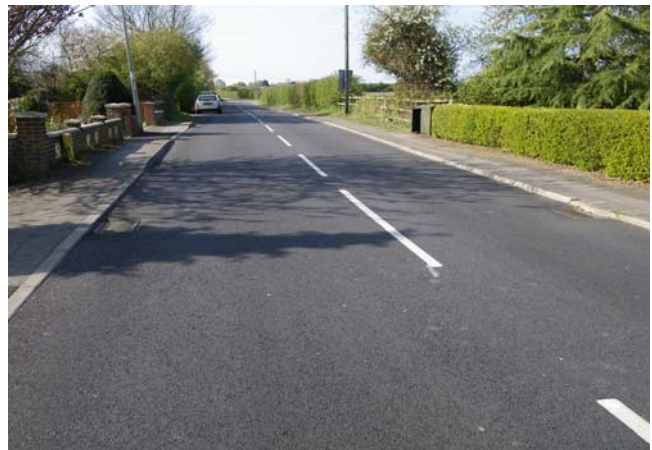
Fig 4:- Vegetex material, New Road leaving the village.
