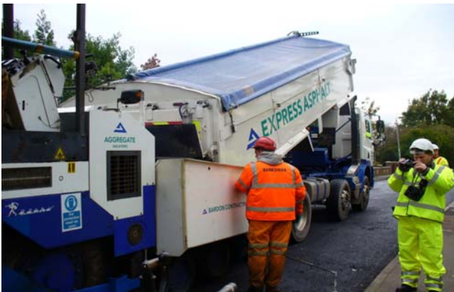
Fig 1:- Laying of AC10 close surf Vegetex 85
