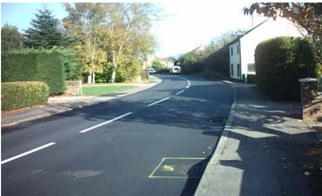
Fig 2:- Compacted AC10 close surf Vegetex 85
