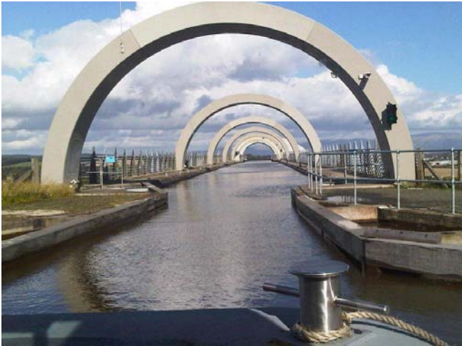
The Elevated Structure of the Upper Canal
