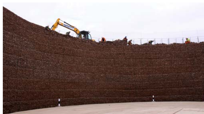
The Gabion Retaining Wall for the Concealment Bunds Nearing Completion
