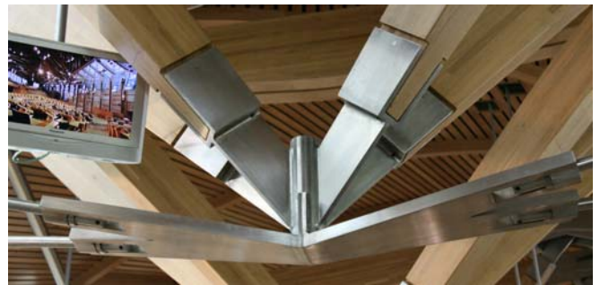
One of the Node Connections
