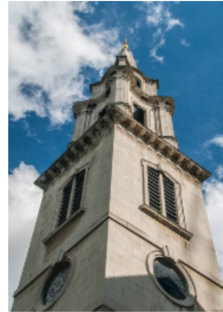
The unusual tower of St Vedast's Church with concave and convex storeys
