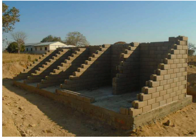
Latrines under construction
