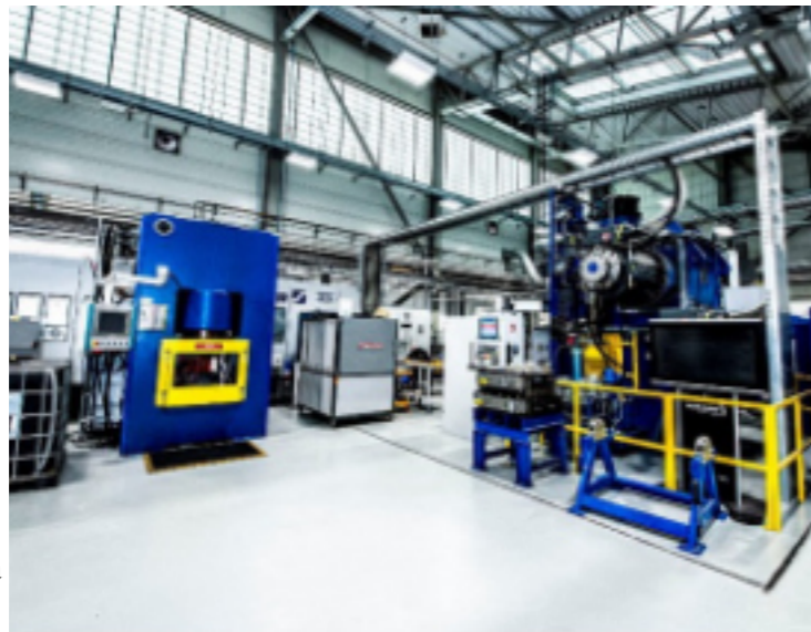
Multi-forge equipment at AFRC
